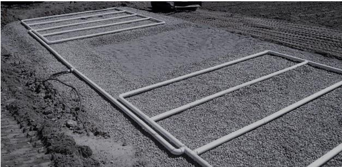
Figure 18. Typical Bed Construction (Partial)
