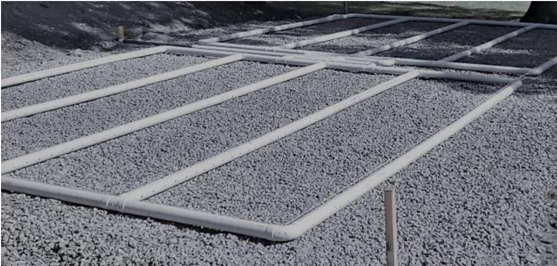
Figure 17. Typical Bed Construction (Partial)
