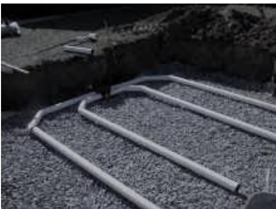
Figure 19. Typical Bed Construction (Partial)
