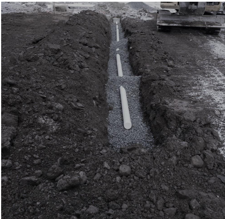
Figure 16. Typical Trench Construction (Partial)
